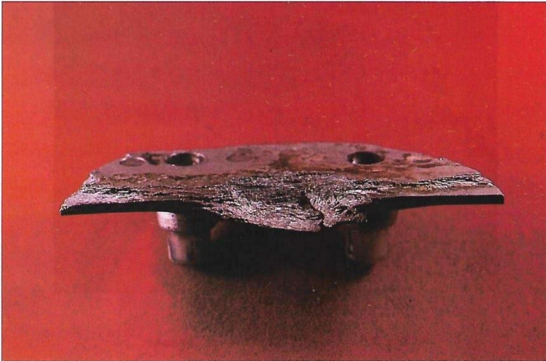
Fig 22 Exfoliation corrosion damage at the edge of an access hole in aluminium alloy skin
