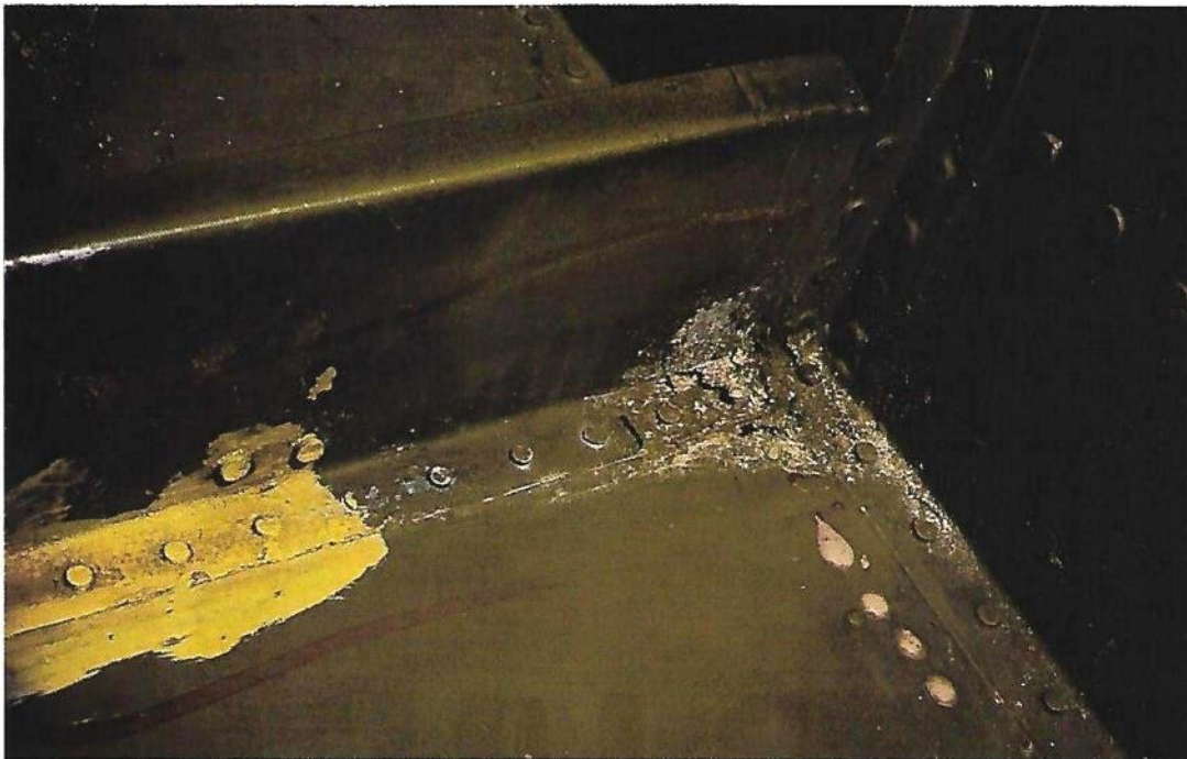
Fig 10 Crevice corrosion between skin and stringer in a Sea King lower fuselage rear bay
