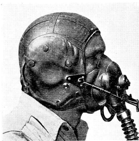
Fig. 7. Oxygen mask, Type A-13A/2— toggle set for pressure breathing
